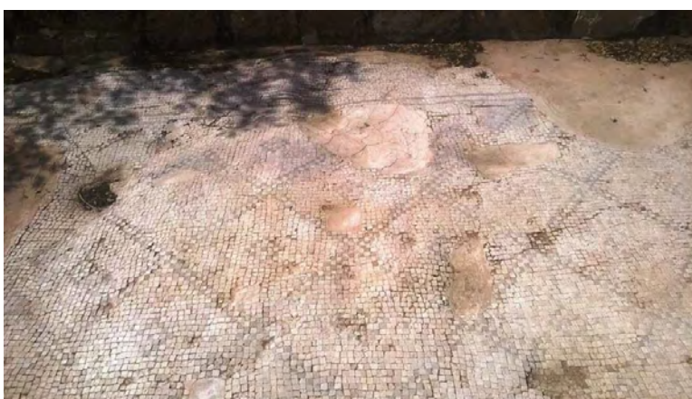
Figure 32. South aisle, first panel
